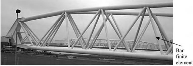
Figure 2.1 A bridge truss.
